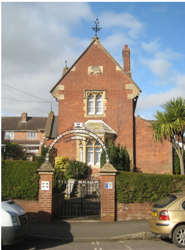
Elevation from street
